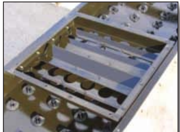
Hot Water Basin Coated with EvapLiner
