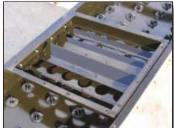
Hot Water Basin Coated with EvapLiner
